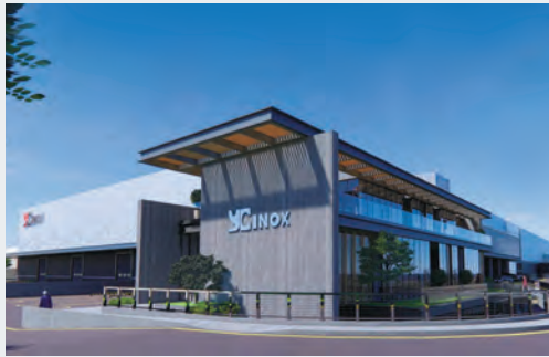
▲ TÜRKİYE PIPE MILL 40,000 m 2
